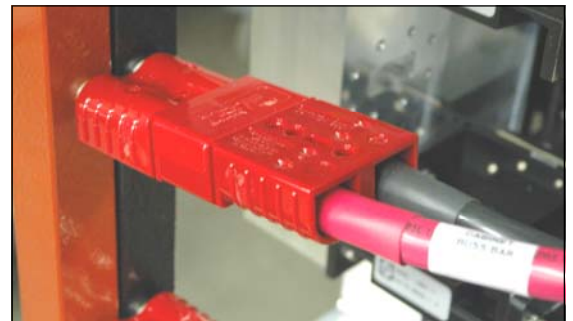
Quick Connect Plug into Bus Rail
